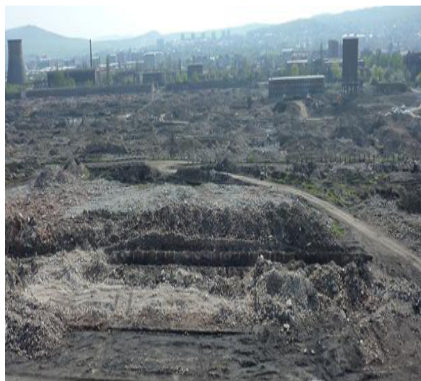
Fig. 10 Area of former iron and steel plant after demolitions of buildings
