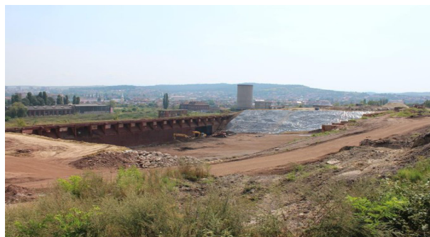
Fig. 9 Former coke-chemical plants area after rehabilitation works
